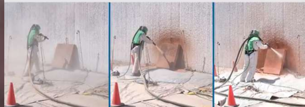
Dry Blasting Water Injection Blasting EcoQuip 2 Vapor Abrasive Blasting
